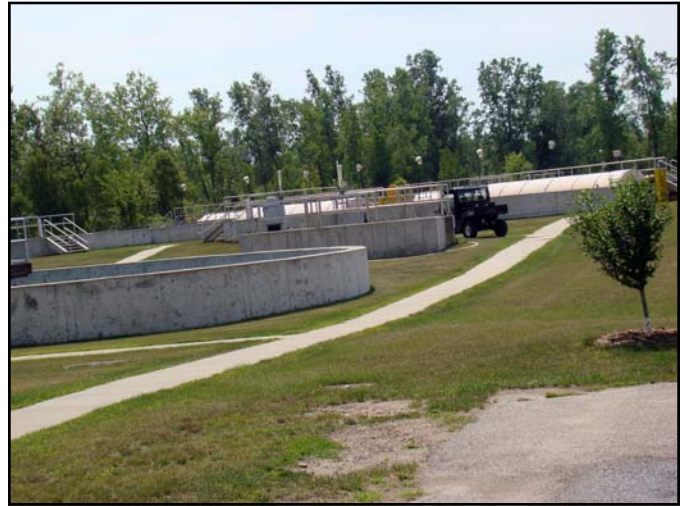
The Waste Water Treatment Plant in Mount Pleasant.
