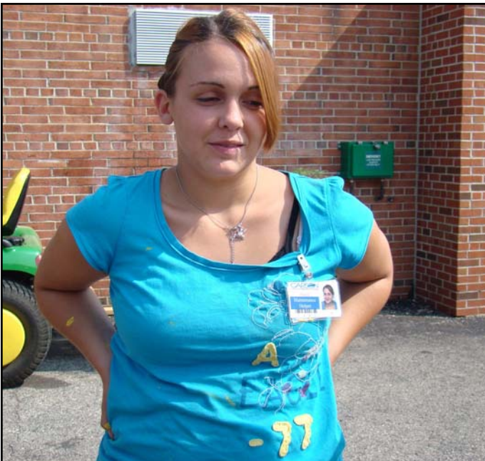
Angela just got done painting guardrails yellow at the Carson City Hospital.
